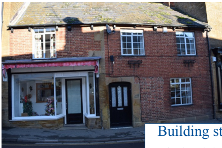
Brick and stone house and shop front, slate roof
