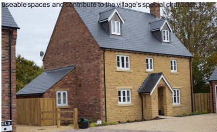
New dwelling at Hayes End showing ample parking space and level access from parking
