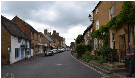
View of St James' Street from the Post Office showing traditional and varied shop fronts; hand painted shop signs; variation in roof heights; and largely 2 storey buildings.
